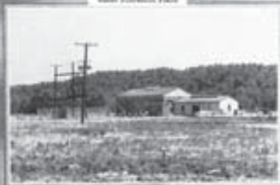
Water Filtration Plant
