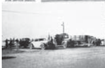
Post Service Station
